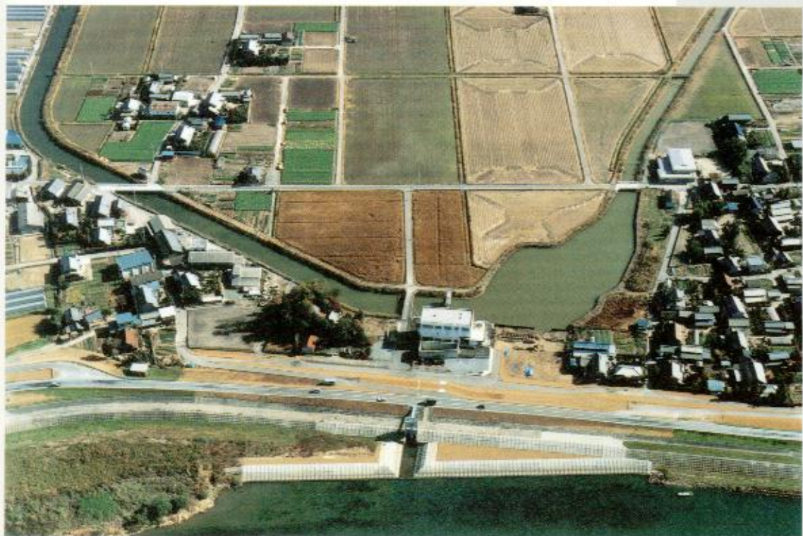
Pump station and drainage canals
