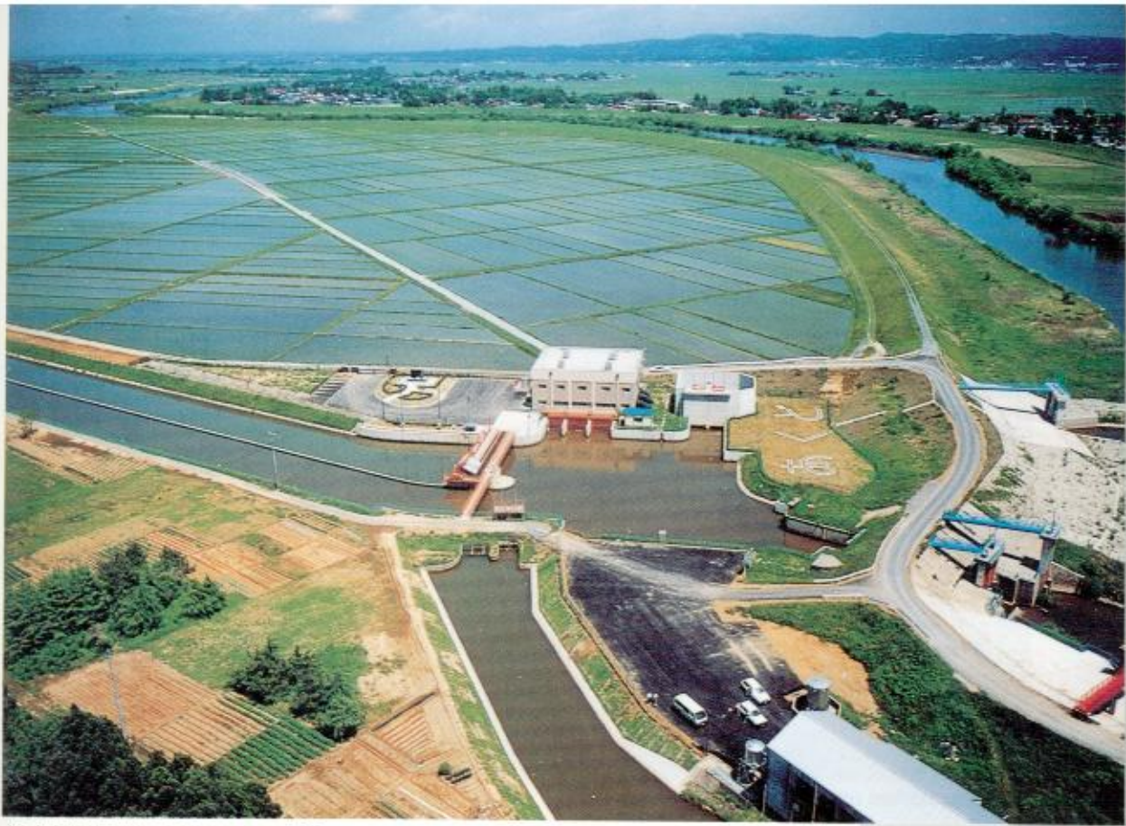
An inland drainage pump station
