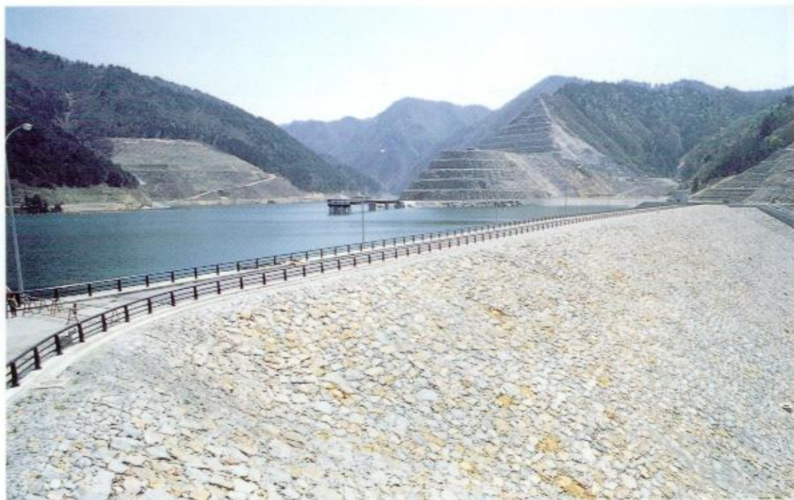
A rock fill dam (close-up)
