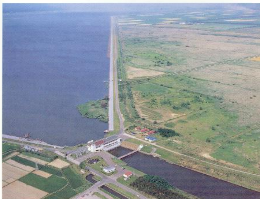
A pump station
