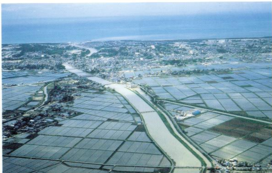
Top center : Shinkawa pump station at the river mouth
