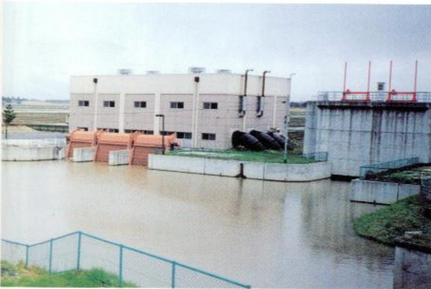
An inland drainage pump station(close-up)
