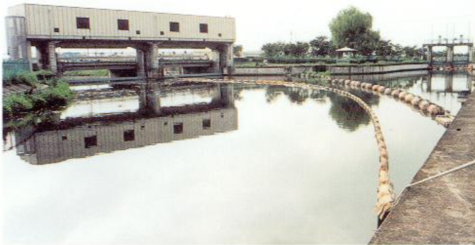
Left : Canal spillway with gates Far right : Check gates
