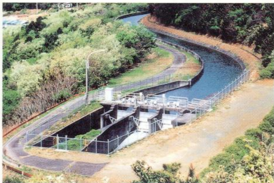
Division or distribution facilities
