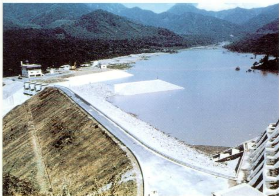
An earth dam (close-up)
