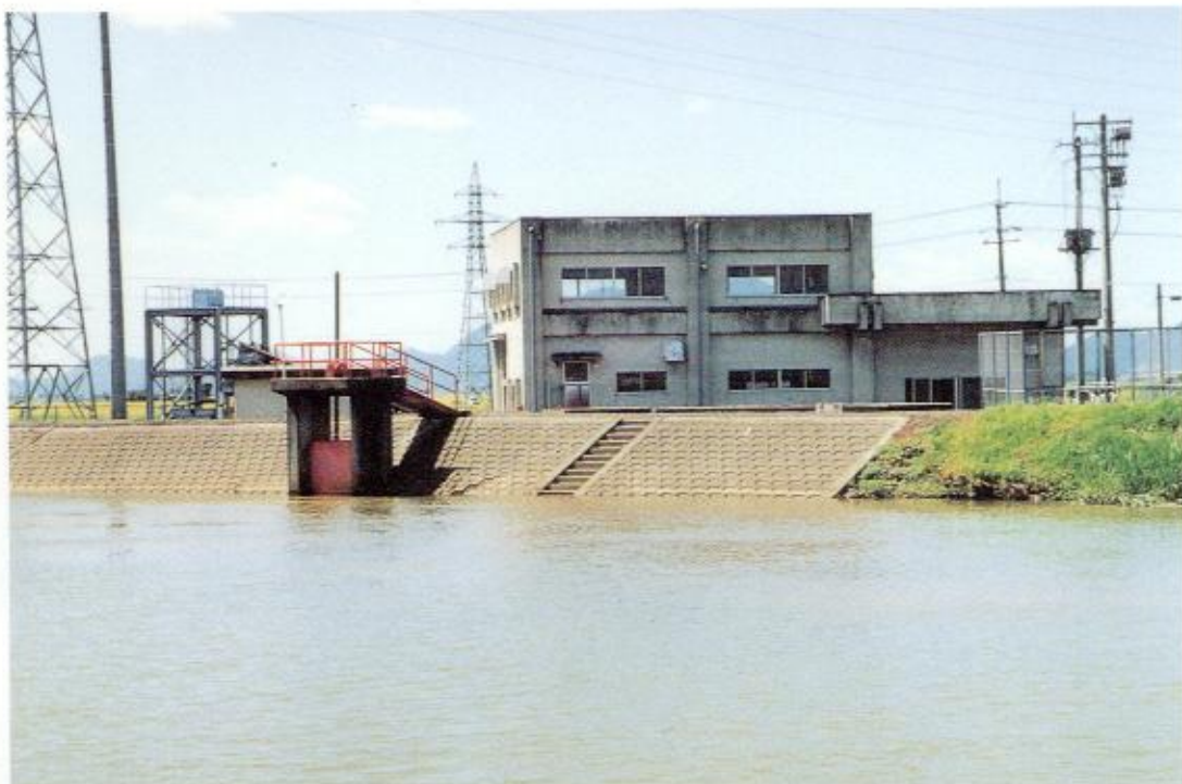
A pump station (river side)
