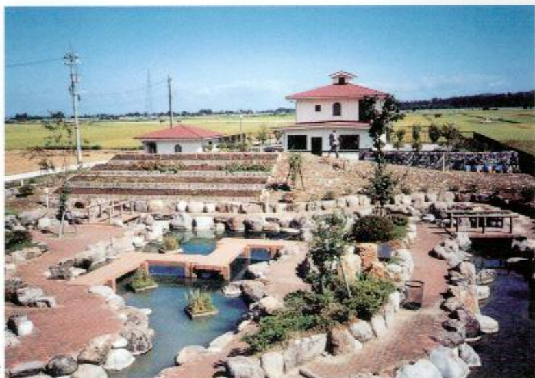
A sewage treatment plant
