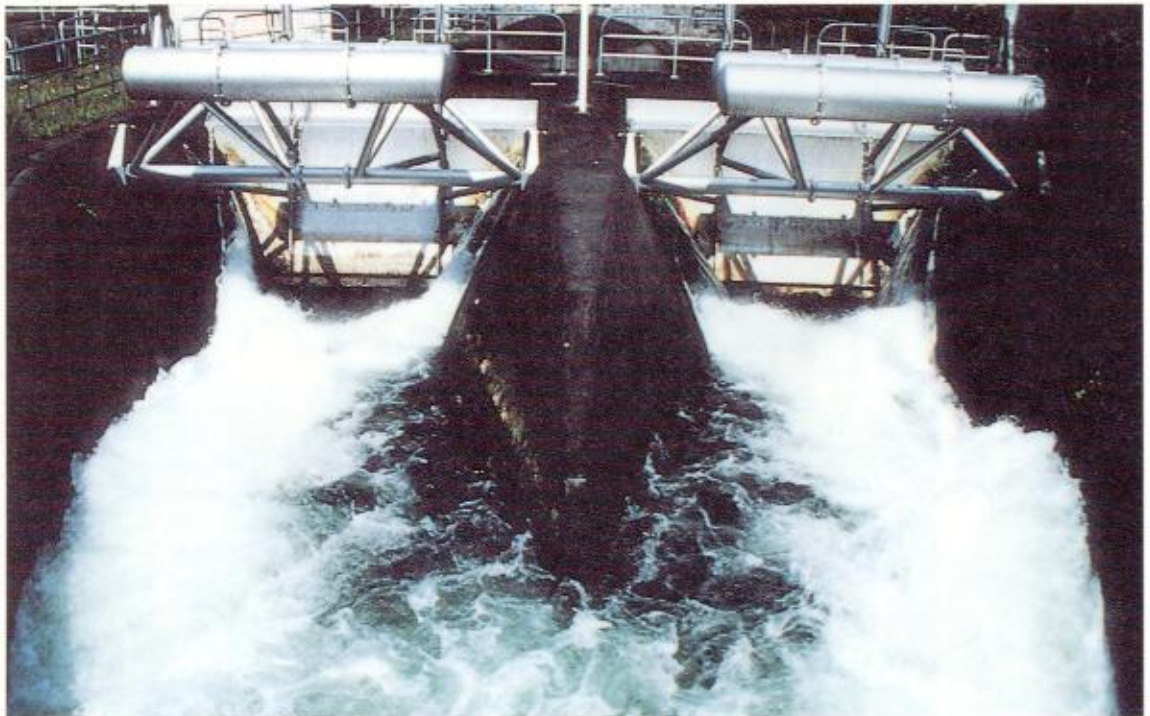
Canal facilities for control (close-up)
