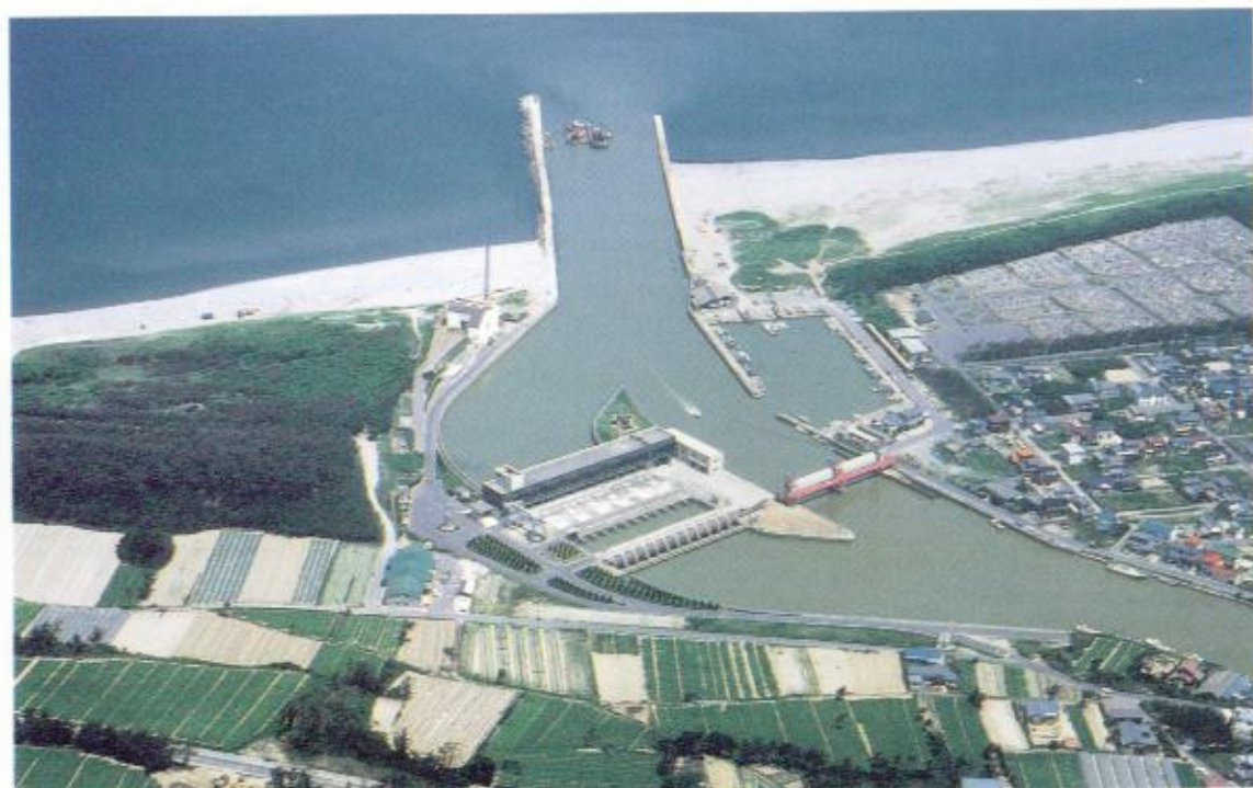
Shinkawa pump station (close-up)
