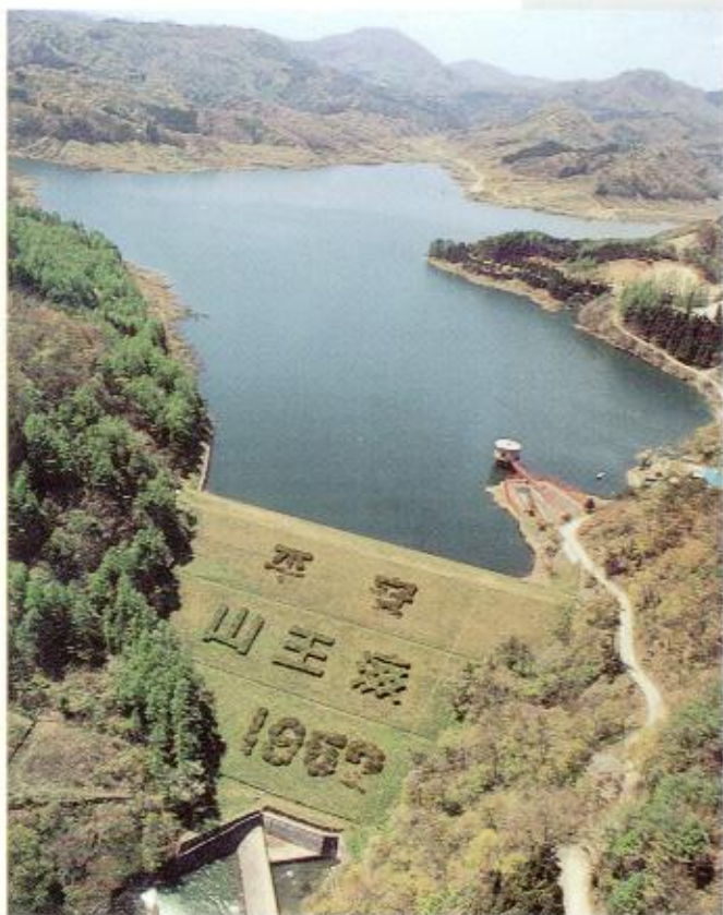
An earth dam
